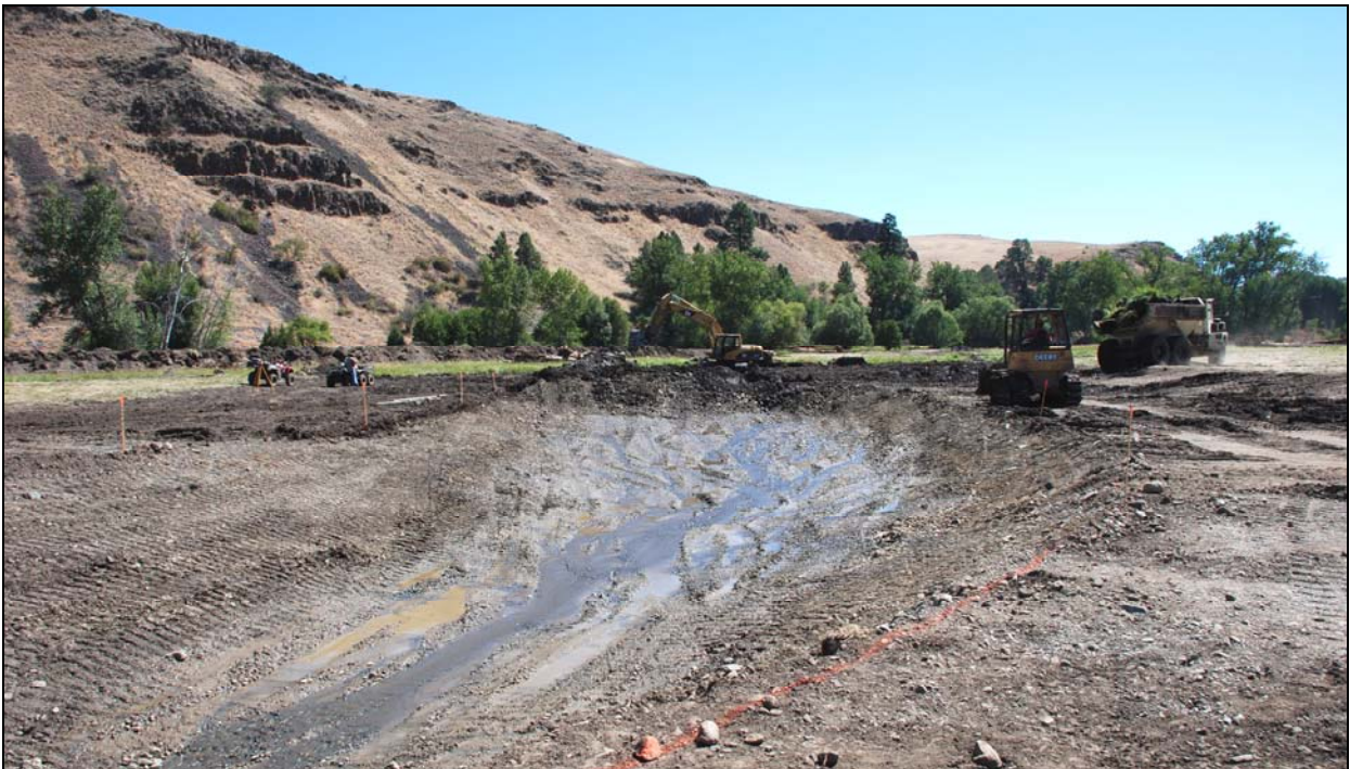
Figure 7. Wallowa River/McDaniel Reach 7a, Ppt. 2, August 2, 2007. LD Perry Construction crews complete the initial excavation of the channel and floodplain cuts.
