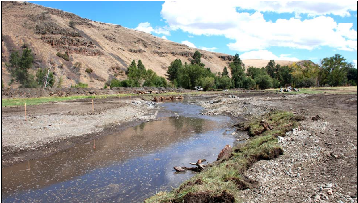
Figure 8. Wallowa River/McDaniel Reach 7a, Ppt. 2, August 21, 2007. Phase I of construction is completed illustrating sedge/rush transplants placed along a rootwad revetment bank. This technique provides lateral channel stability (prevents erosion of the near bank) as well as complex hiding cover for fish. The channel has not yet been connected (scheduled for 2008), but groundwater seepage has begun filling the pools.
