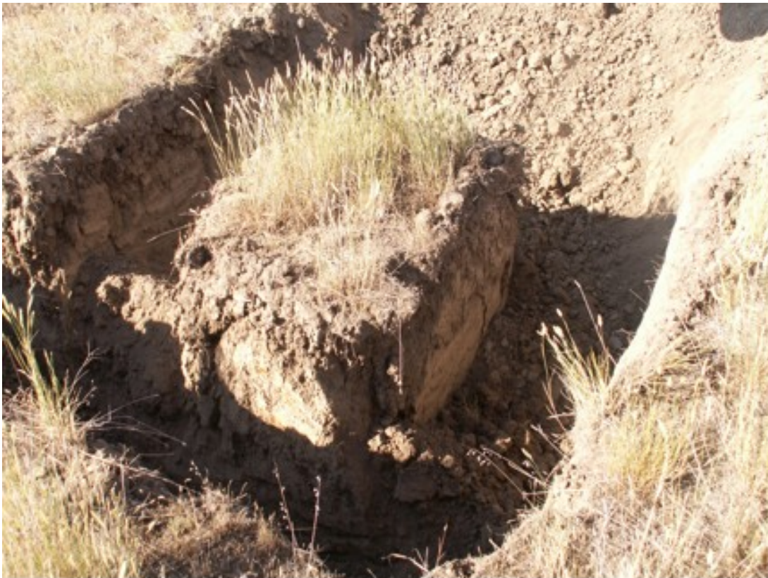
Figure 7.5: Excavation of the soil monolith to be placed on the drainage gauge lysimeters.
