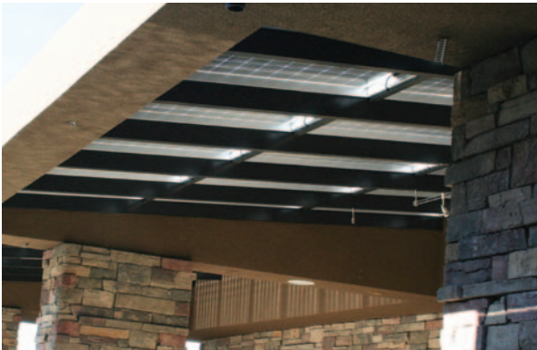
Bifacial solar panels receive sunlight from above and below simultaneously, converting it to electricity.
