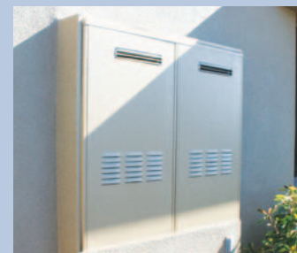
High-efficiency tankless water heaters save heating energy and provide ample amounts of hot water.
