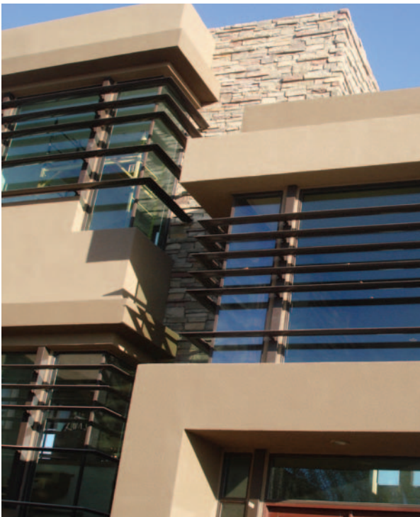
Horizontal louvers extend across the windows to provide shading.
