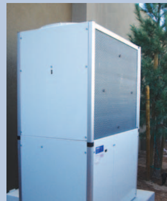
The gas-fired heat pump efficiently provides heating and cooling to the home.
