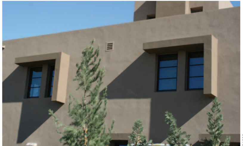
Eyebrows integrated into the walls block the intense rays of summer's late afternoon sun.
