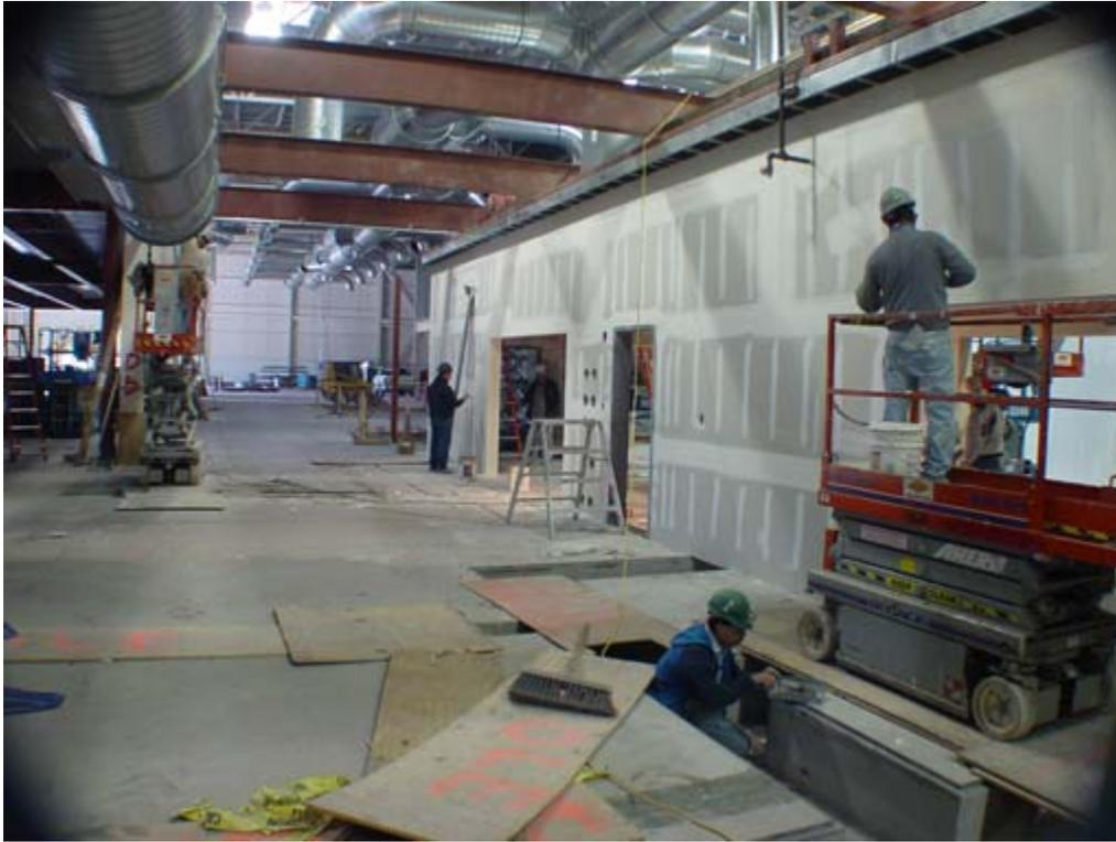
**Fig. 7** Interior structures, equipment chases and HVAC under renovation in the Tucson facility.
