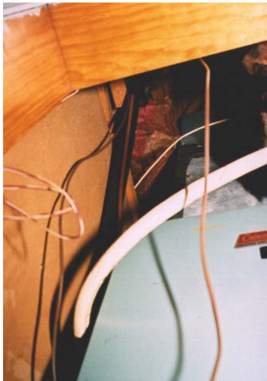
Figure 3.2. Unsealed equipment chase permits infiltration.
