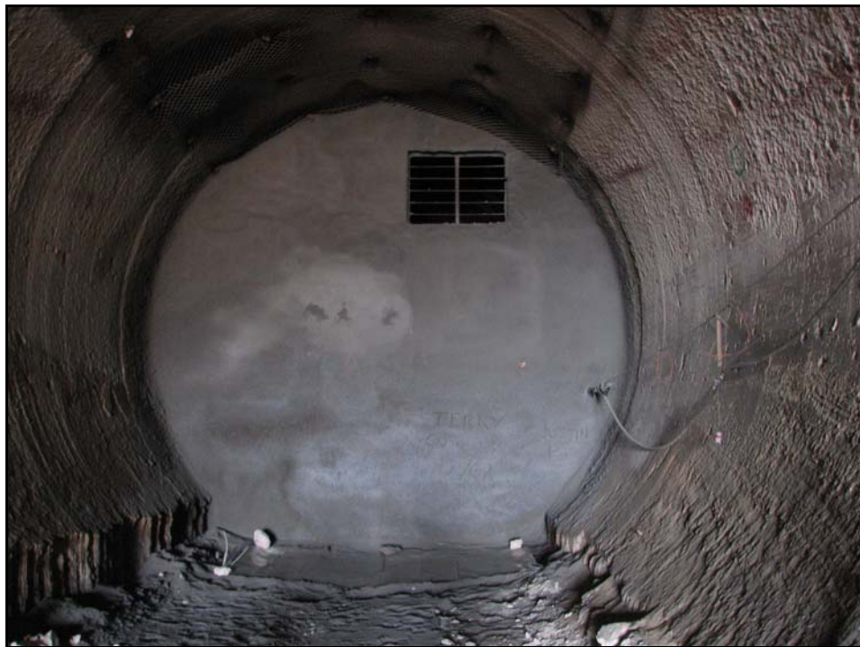
Figure 6-18. Completed bat gate in the extension drift of N Tunnel with plastic sheeting on ground below (Photo taken by D. B. Hall, February 8, 2007)
