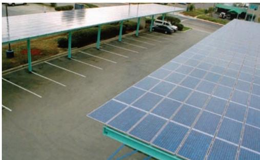
*The City’s first PV system is a 62-kilowatt (AC) carport array at the ESD Operations Center.*
