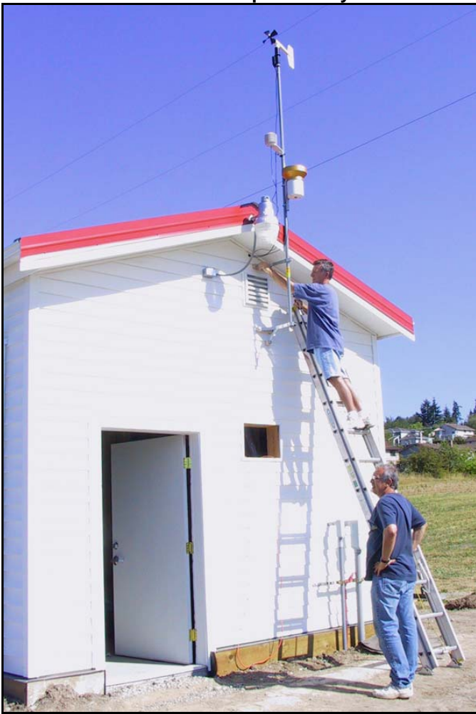
9 Installation of the weather station
