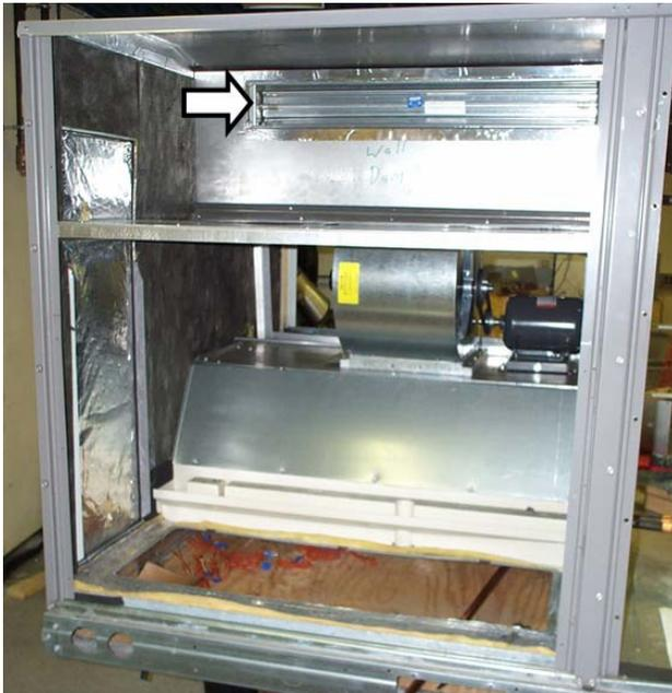
**Figure 16: Outdoor Air Throttling Damper**
