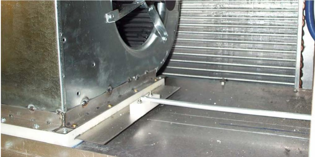
**Figure 15: Return Blower Discharge Damper**
