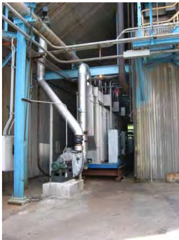
Photo 6-B. Gas ID Fan and Pilot ESP
