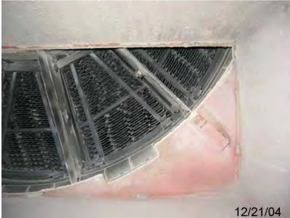
Figure 46. Cold End Basket After Soot Blowing
