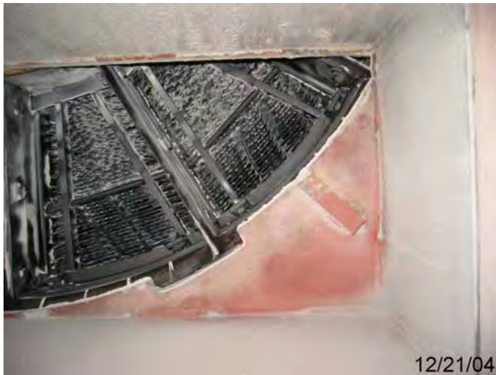
Figure 45. Cold End Basket Before Soot Blowing
