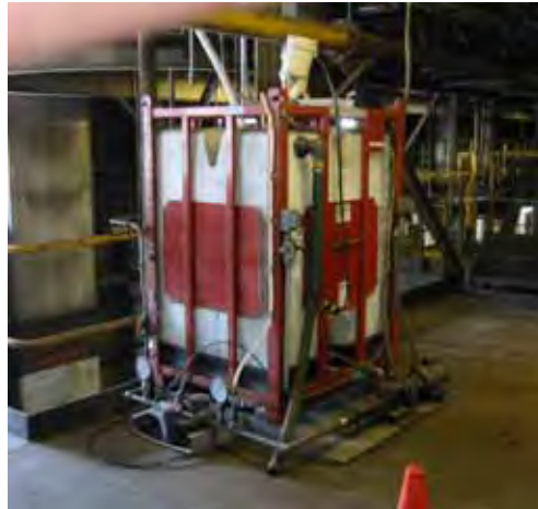
Photo 1-B. Dilute Slurry Day Tank with Agitator, Circulation Pump and Filters
