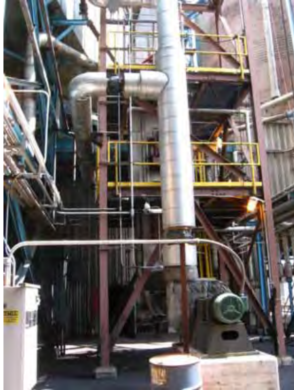
Photo 4-B. Flue Gas By-Pass Fan with Tee-In for Pilot ESP Gas, Pilot Air Heater in Tower Behind
