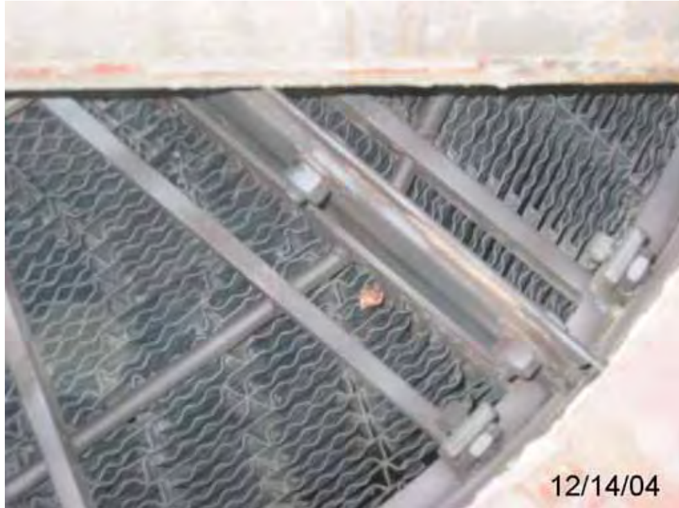
Figure 41. Cold End Basket After Soot Blowing
