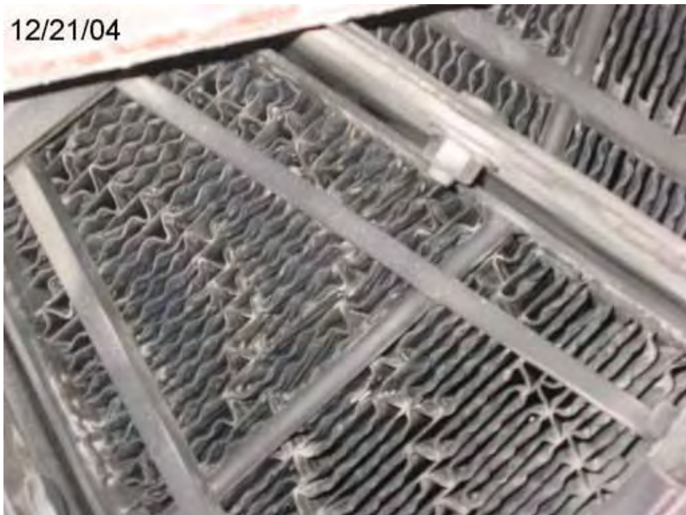
Figure 47. Cold End Basket After Soot Blowing
