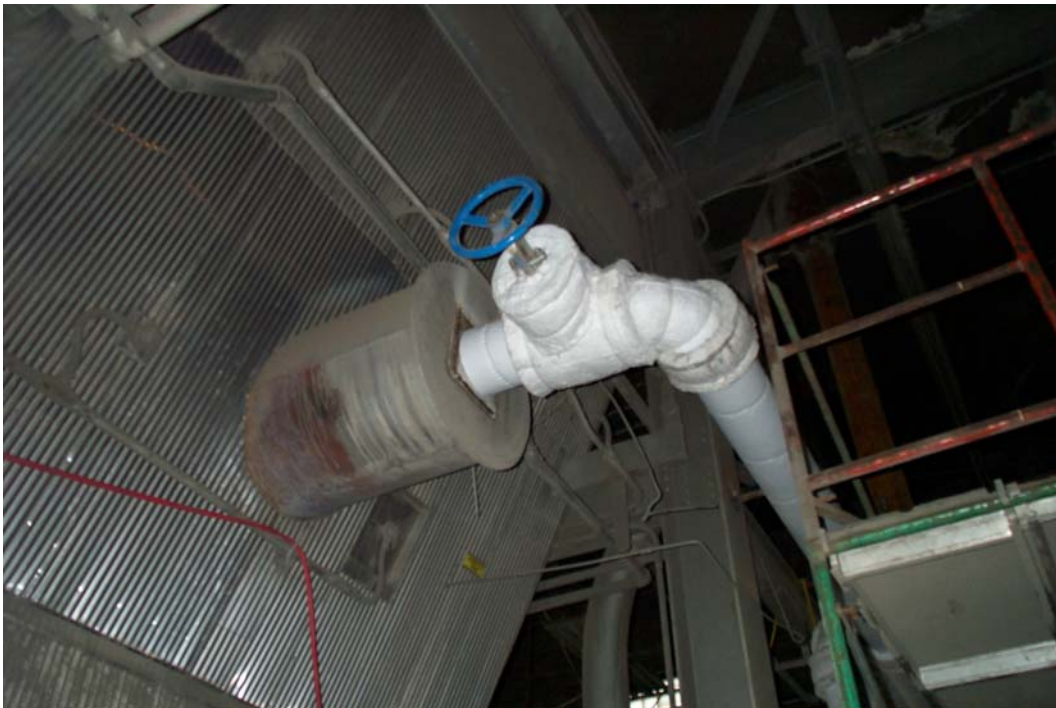
Figure 12. Outlet port located downstream of air heater.
