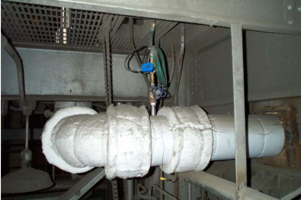
Figure 11. Inlet port located upstream of air heater.
