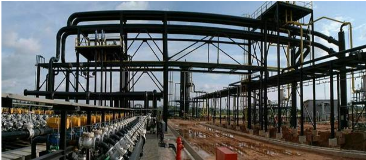
Figure 25 – Dual GLCC ® -Slug Damper (SD) System Installed in the Field in Indonesia (Courtesy: Chevron)
