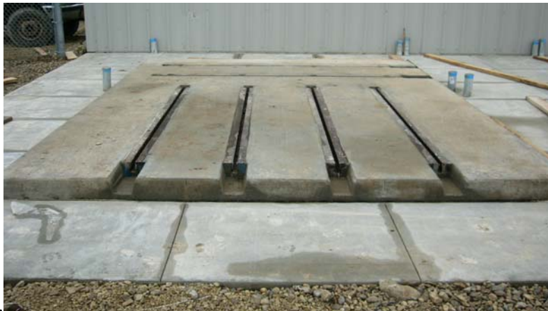
Figure 1. Completion of engine base.
