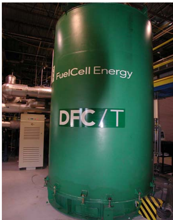
Figure 1. SubMW DFC/T HYBRID POWER PLANT FACILITY: Full-Size DFC Stack Was Integrated With Capstone C60 Microturbine
