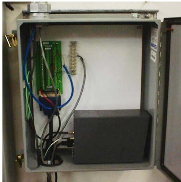
Figure 13. Control cabinet for cylinder pressure monitoring system
