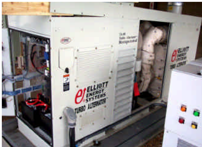
Elliott microturbine (80kW) opened for servicing
