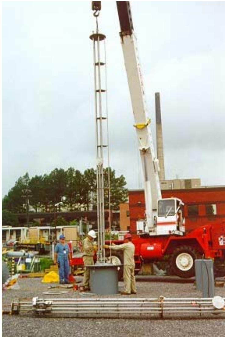
Fig. 2. PulsAir Mixer during installation at GAAT W-9.
