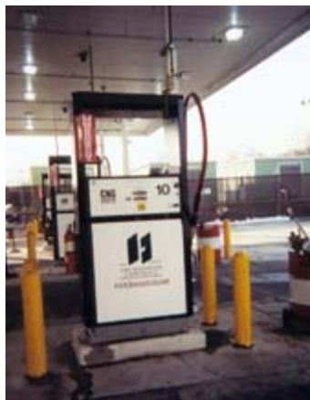
Figure 7. CNG Fueling Dispenser at WMATA
