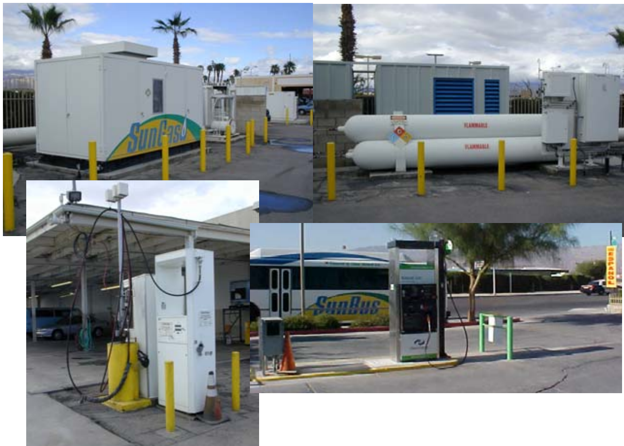
Figure 8. CNG fueling equipment (Indio)
