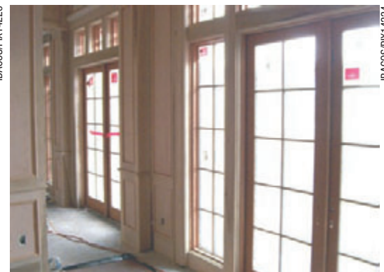
High-performance windows with impact resistant properties were installed throughout the home to limit solar heat gain.
