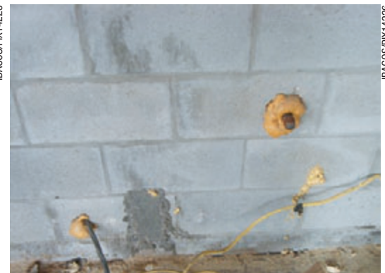
All openings and penetrations are sealed to keep the home airtight and prevent moist hot air from entering the house.
