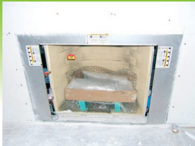
Three propane, direct-vented fireplaces guide smoke away from the house.
