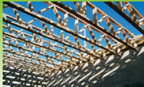
Installing open-web floor trusses requires careful structural integration with the block wall construction.
