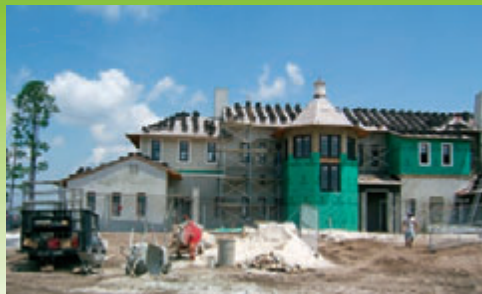
Installation of housewrap provides a drainage plane, which prevents moisture problems.
