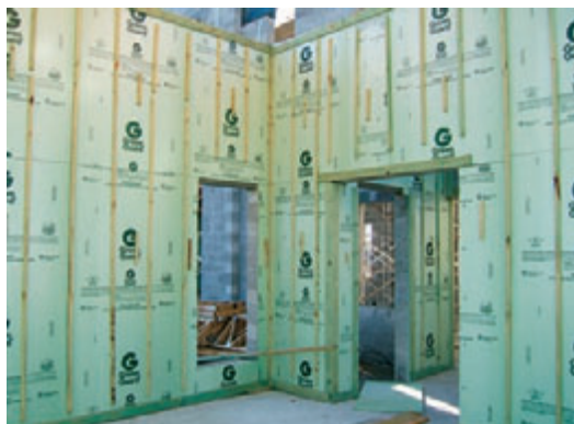
R-5 extruded polystyrene panels are mounted continuously inside the exterior walls, contributing to the home's insulation qualities.
