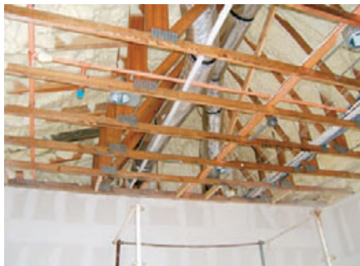
The use of spray-foam insulation underneath the roof deck offers a more hospitable area for ductwork and air handlers by turning the attic into a sealed, unvented, and conditioned space.
