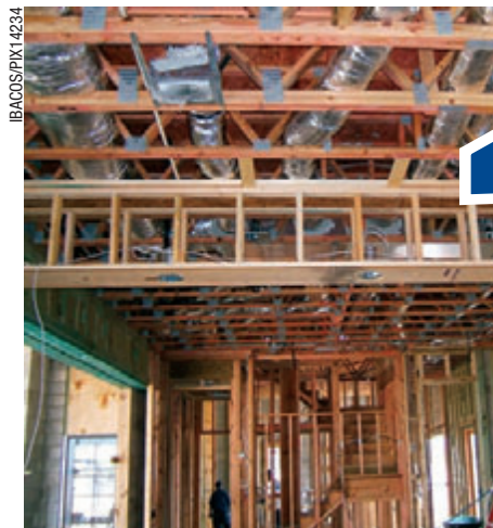
Open-web floor trusses eliminate obstructions, allowing efficient installation of ductwork and other services.
