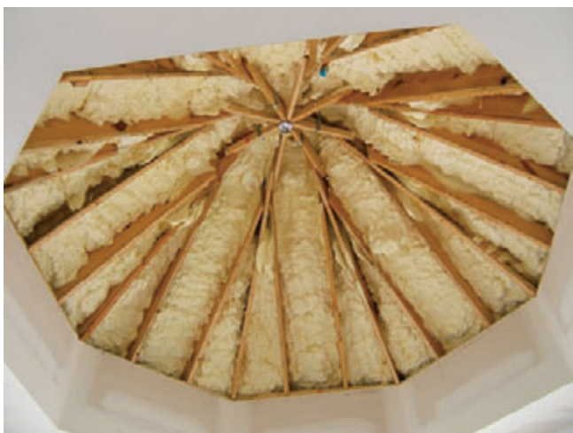
Spray-foam insulation was carefully installed in the top of the two-story entrance tower to prevent air movement and to insulate the home.
