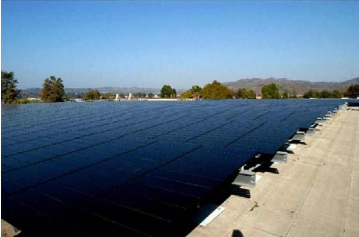
**Figure 43. SSI's new 245 kW CIS thin film array.**
