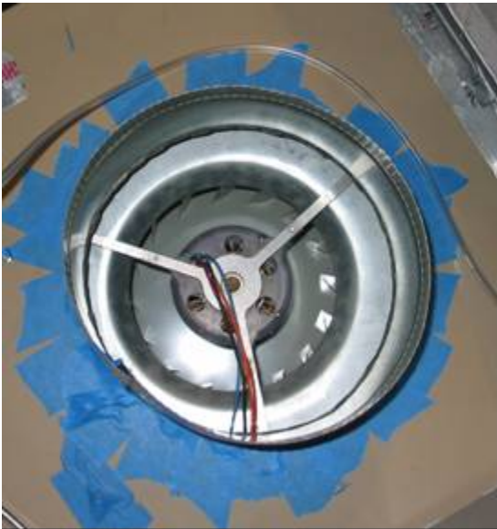
Figure 10. Fabricated Motor Side entry for Furnace #1
