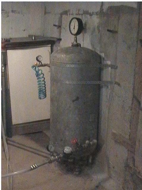
Figure 10. Pressurized water tank (1) with pressure gauge p_1 on top.
