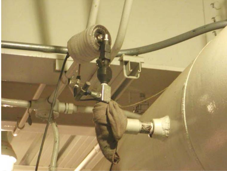
**Figure 4-9. Heated Pressure Sensor (Discharge Lateral); Dresser-Rand TCVC10; Dominion Groveport Station Unit 1; April 20, 2005**
