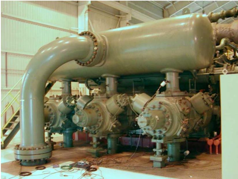
**Figure 4-2. Heated Pressure Sensors Temporarily Installed on Cylinder 1; Dresser-Rand TCVC10; Dominion Groveport Station Unit 1; April 20, 2005**
