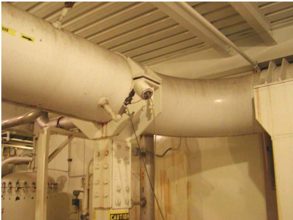
**Figure 4-8. Heated Pressure Sensor (Suction Lateral); Dresser-Rand TCVC10;
