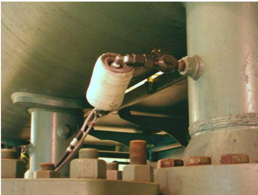
**Figure 4-4. Heated Pressure Sensor Installed on Suction Nozzle; Dresser-Rand TCVC10; Dominion Groveport Station Unit 1; April 20, 2005**
