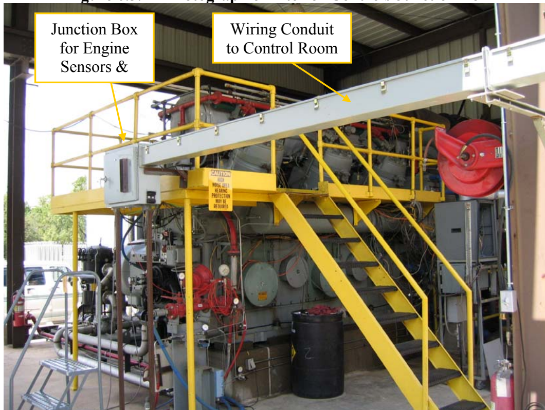
Figure 6.4. Photograph of Engine-Side Control Junction Box
