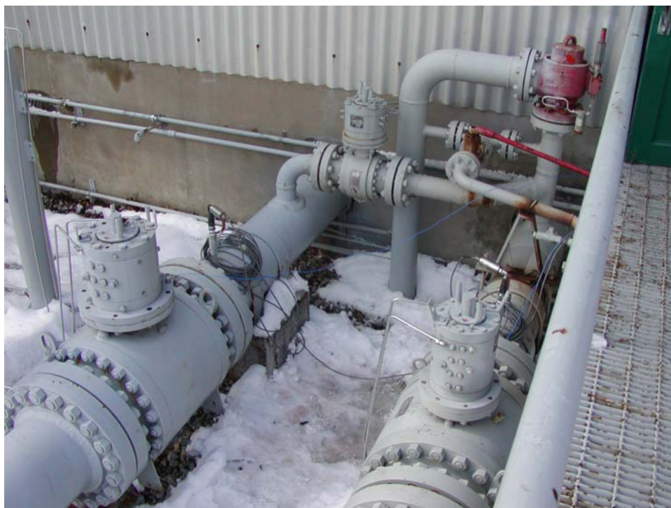
Figure 4-4. Installation of Header Pressure Transducers; Clark HBA-6 Unit 4 (Duke Energy's Bedford Station; March 1, 2005)
