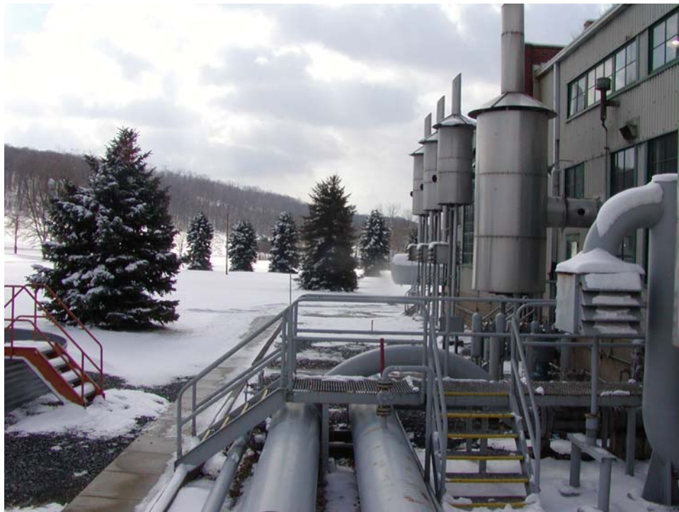
Figure 4-1. Photograph of Compressor Building Showing Unit Stacks (Duke Energy's Bedford Station; March 1, 2005)
