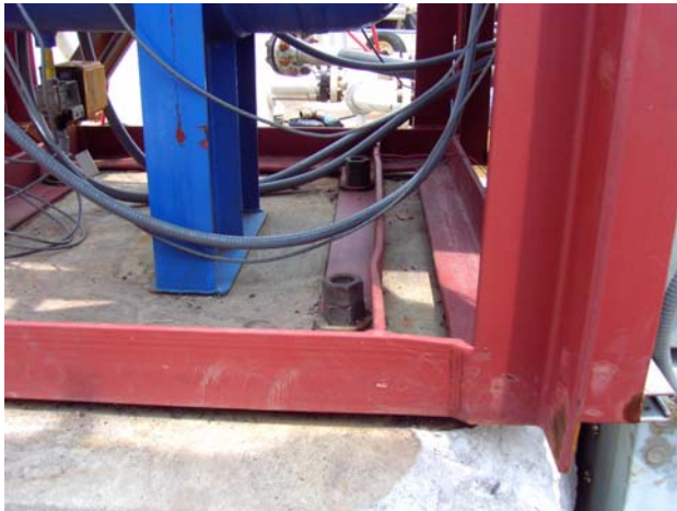
Fig. 2.4 Deformed mast support structure
