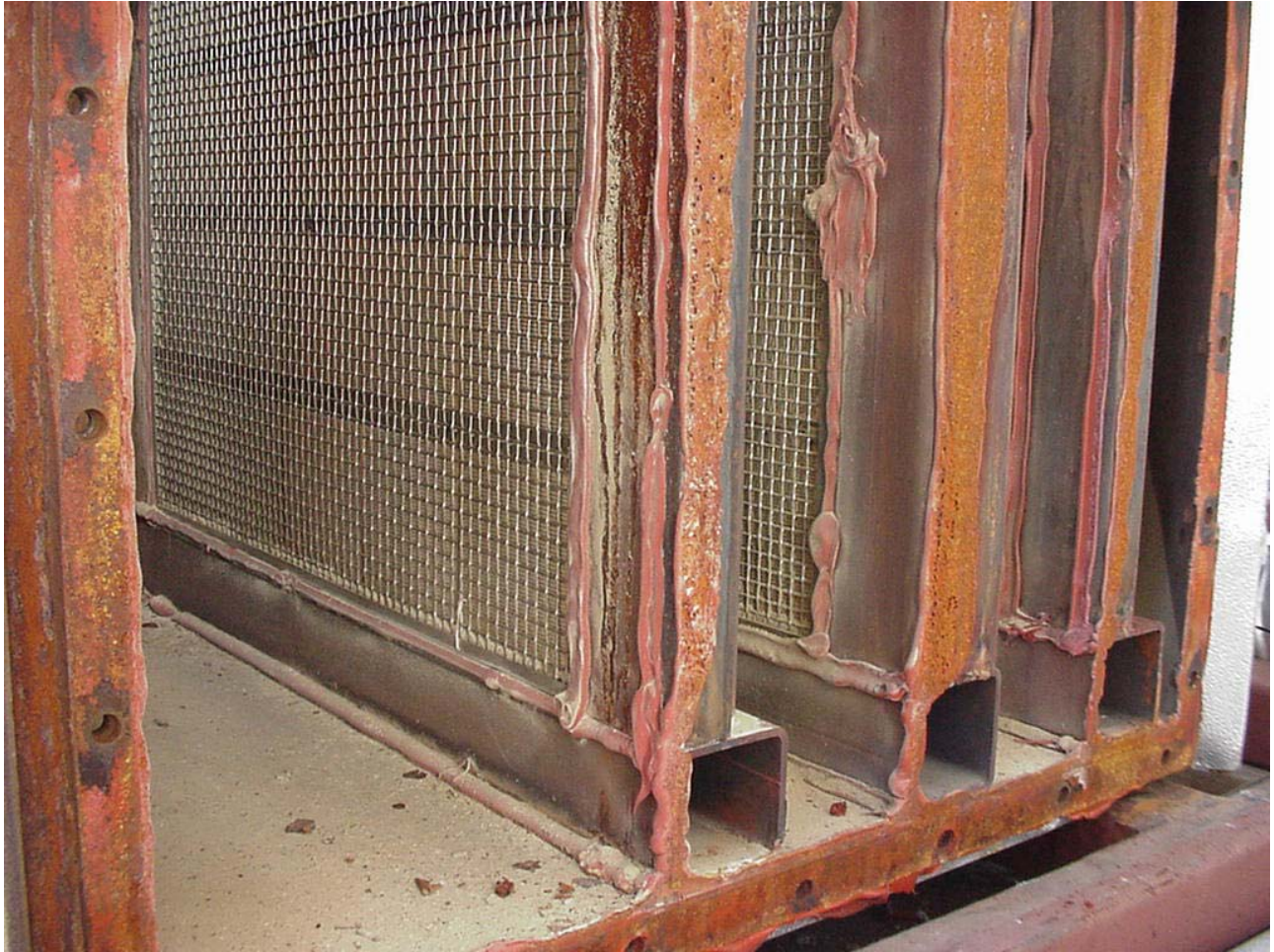
Figure 5. Photograph of a Catalyst Chamber at Spruce Showing Minimal Fly Ash Buildup after One Month of Operation
