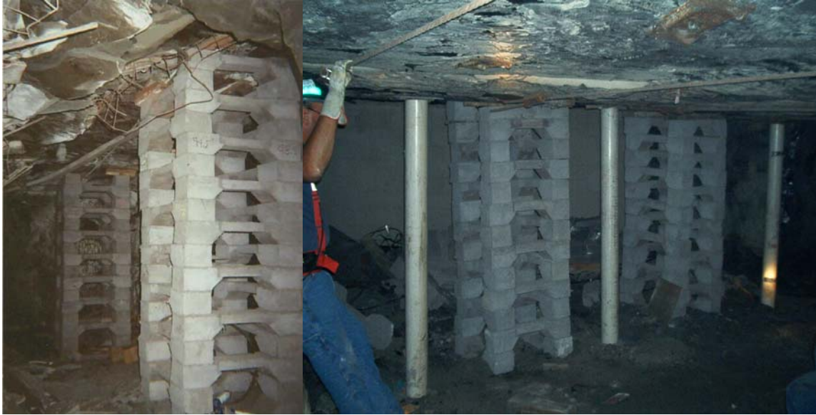
Figure 39: Installed Cribs at Mine # 1 and Mine # 2
