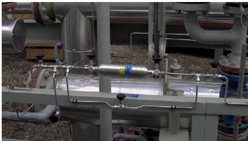
Figure 7. Typical Sampling arrangement at sample location
