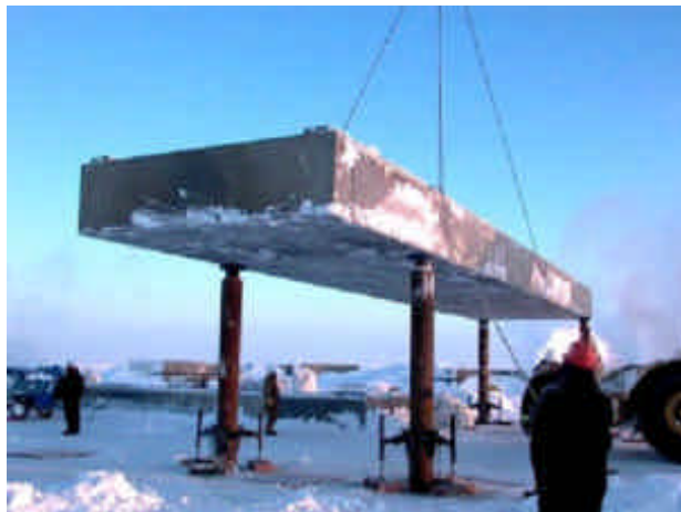
Figure A-3. Setting the First Platform Module
