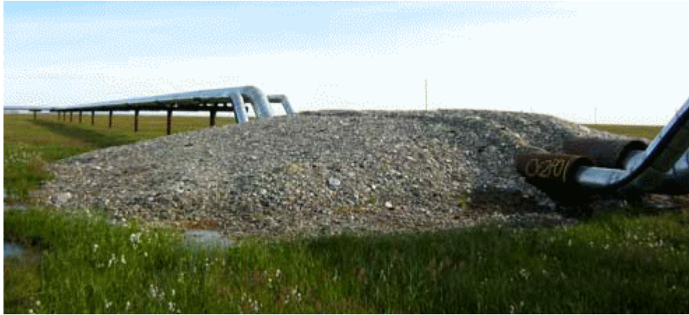
Figure 8. Gravel Ramp for Pipeline Crossing
