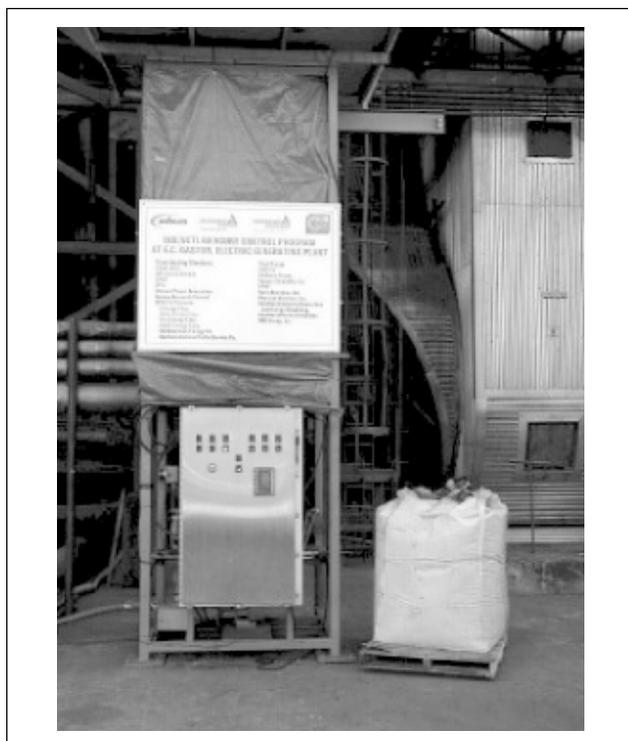
**Figure 2.** Carbon injection skid installed at Plant Gaston.
