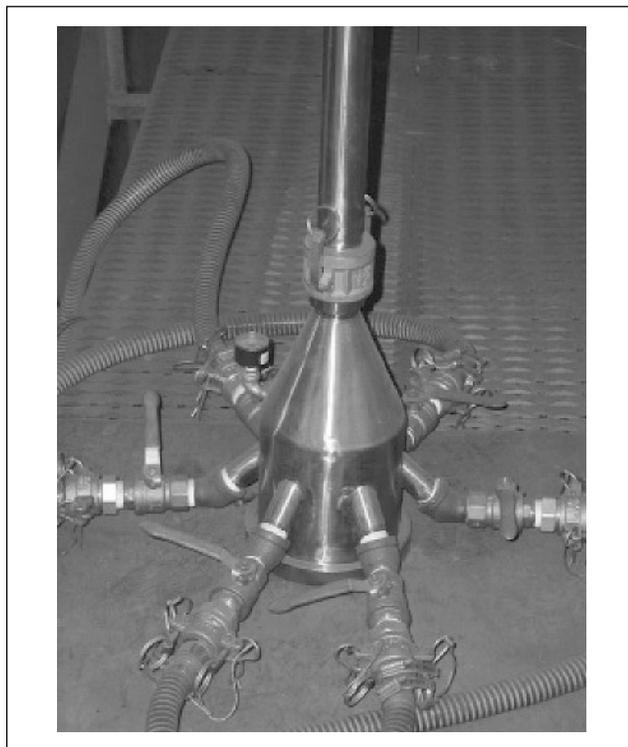
**Figure 3.** Distribution manifold for injection lances at Plant Gaston.
