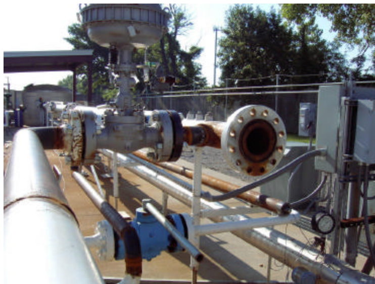
Figure 3.2 – Piping to Drill Section Re-routed to Accommodate Rotation System
