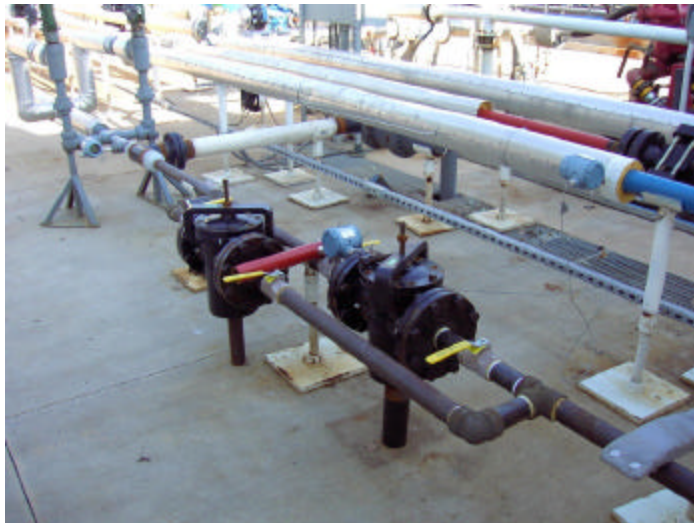
Figure 3.7 - Installed Strainers
