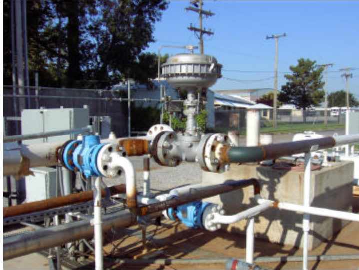
Figure 3.1 – Piping Changes to Accommodate Rotation System
