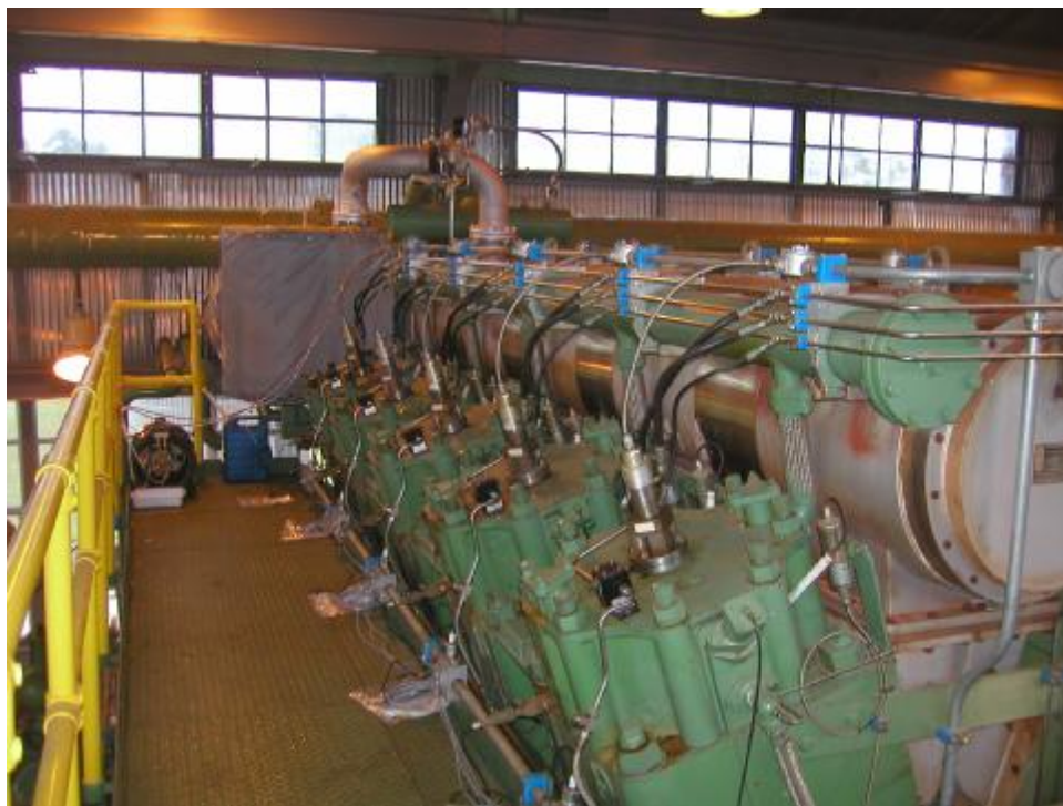
Figure 4-2. Power Cylinder, Left Bank
