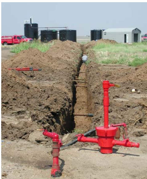
Figure 2. Laying fiberglass injection line from the water supply plant to the CO2#10 water injection containment well. View is looking to the northwest.
