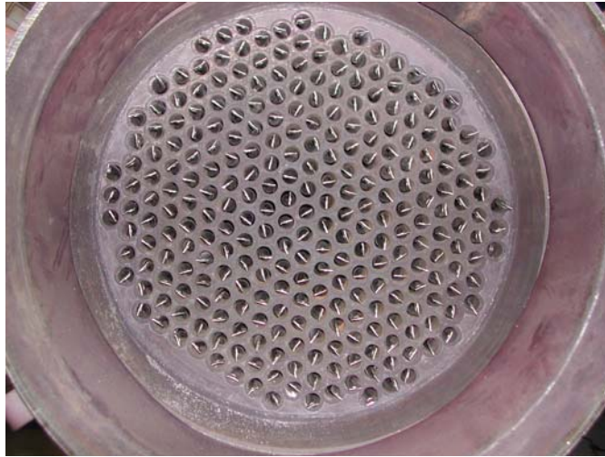
Figure 3. Twisted Tape Wire Inserts Installed in HEX 370
