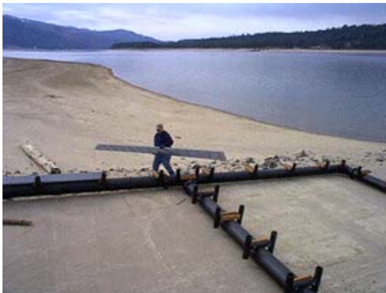
Expanded plastic decking being put into place on pen frame
