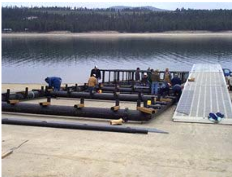
Partially assembled net pen, background pens have the safety handrail installed, fish nets will be installed when pens are floated to locations prior to loading with fish.
