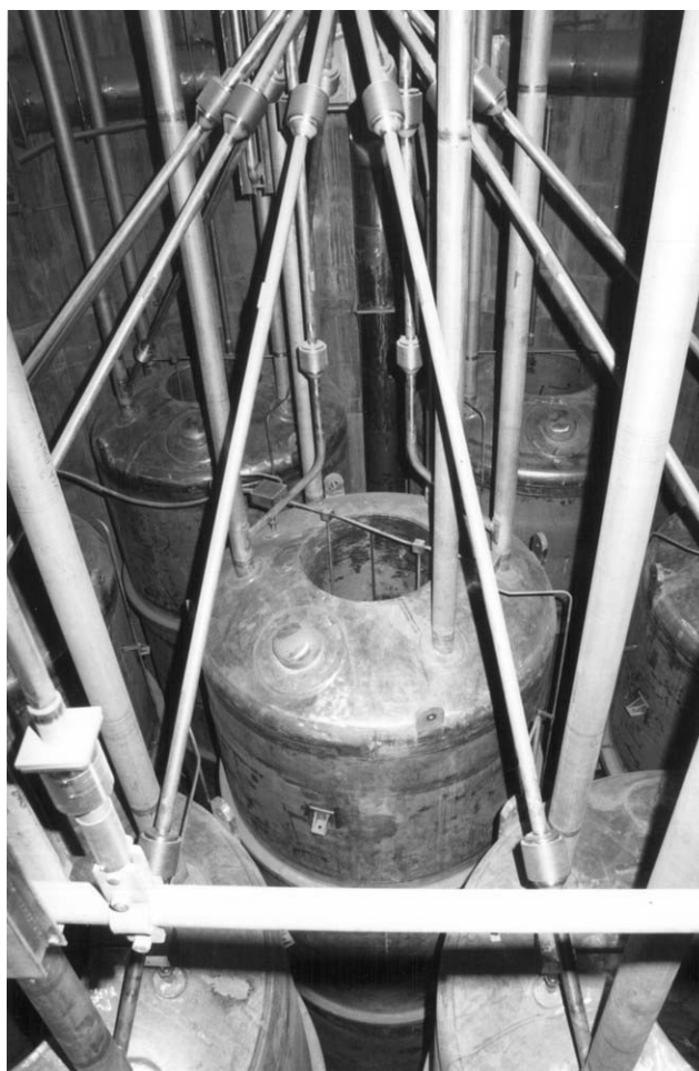
Figure A-7. Distribution piping for Calcine Solids Storage Facility VI (84-680-1-6).
