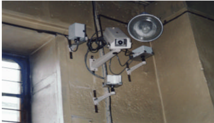
Figure 13. An Example of Remote Monitoring Equipment in a Storage Vault
