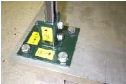
Figure 8: the connection to the base plate
