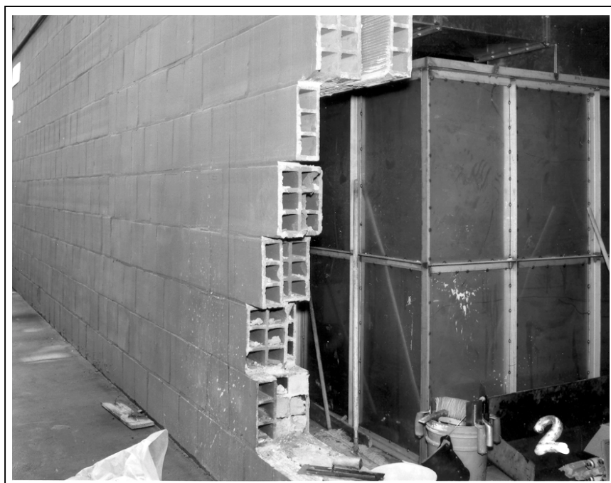
FIG. 1. Section of wall Infilled with Structural Clay Tile
