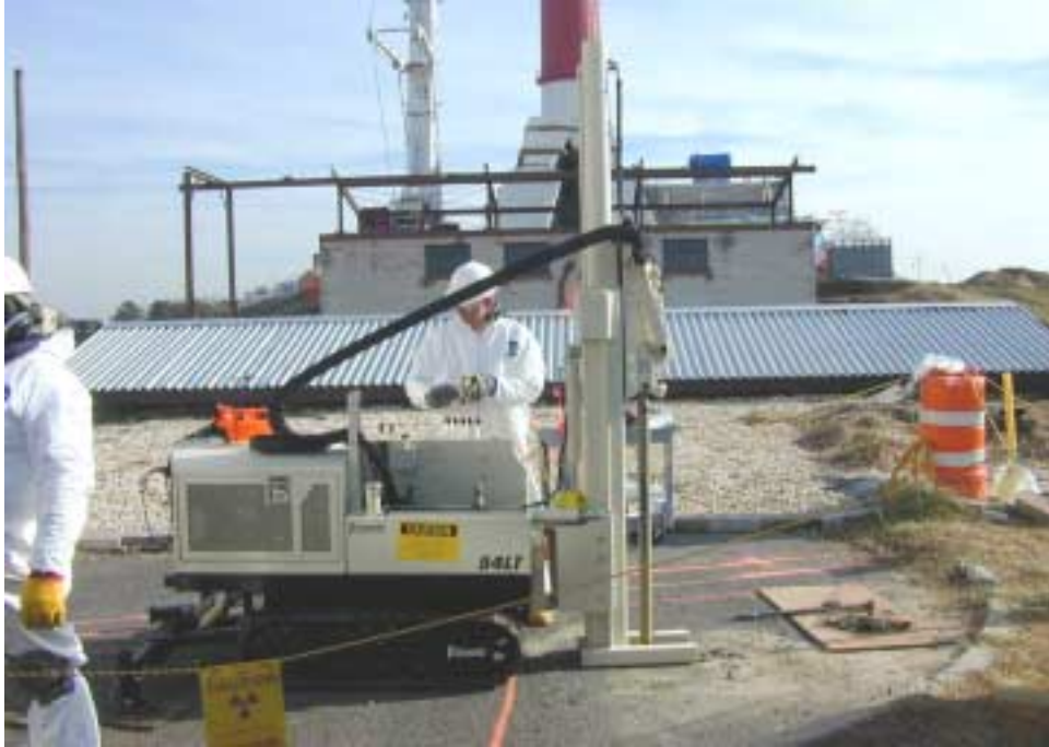
Figure 4. Geoprobe® Model 54 LT continuous push soil-probing unit used to install monitoring ports in soil adjacent to the BGRR Below Grade Ducts
