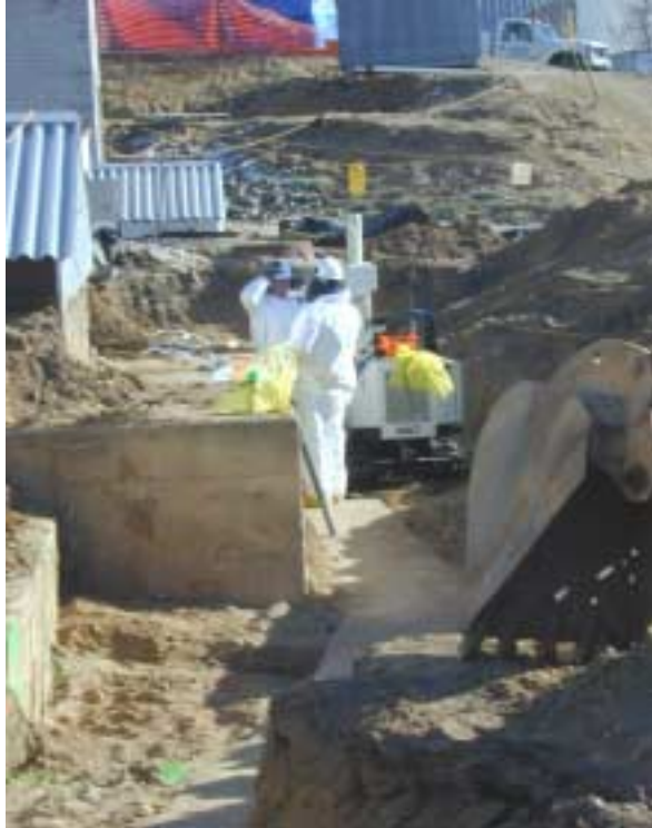
Figure 17. Geoprobe® installing ports along the South Duct, between the electrical duct and the BGD
