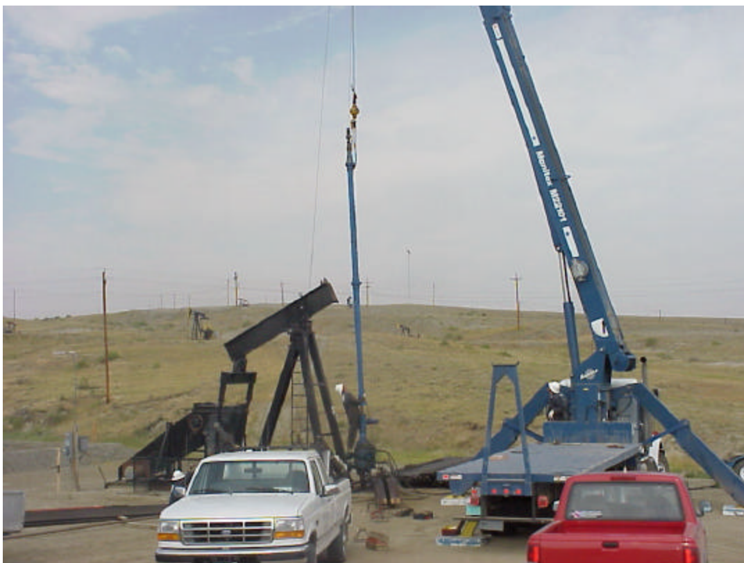
Picture 6. Well 61-A-3. First tool being lowered inside wellhead lubricator and BOP equipment.
