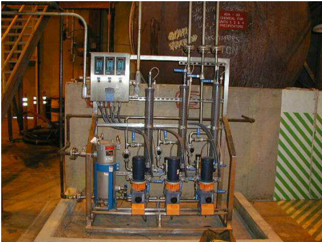
Figure 1: Chemical Metering Skid
