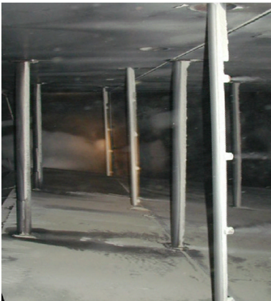
Figure 2: Spray Lances Inside Duct
