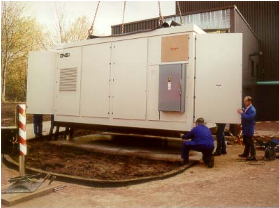
PC25C power plant unloading and installation
