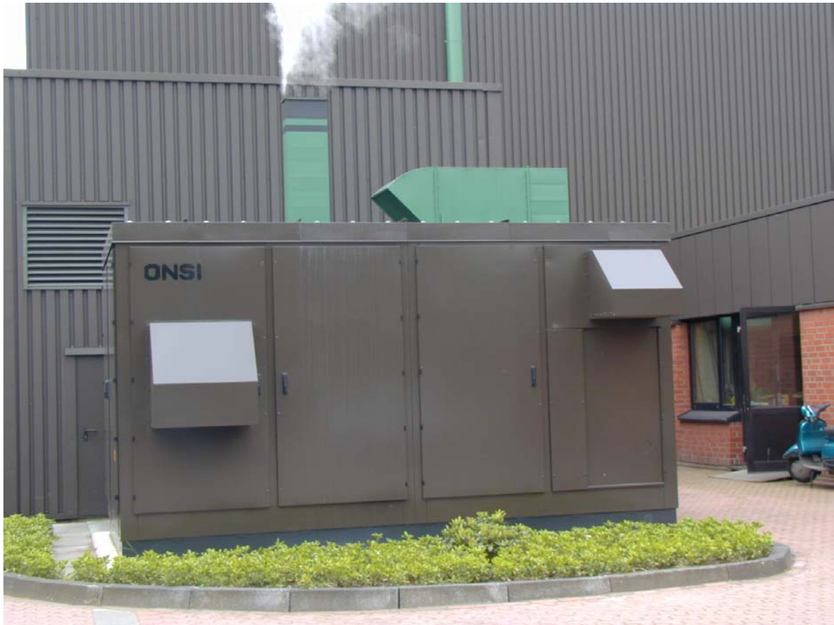
PC25C fuel cell power plant at the St.-Agnes-Hospital in full load operation
