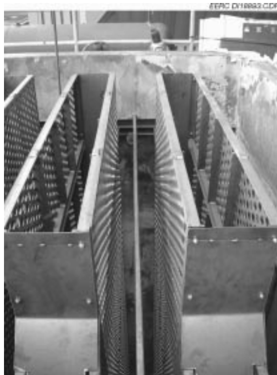
Figure 13. Installing the perforated plates in the 9000-acfm ( 255\text{-m}^3/\text{min} ) AHPC at the Big Stone power plant, March 2001.
