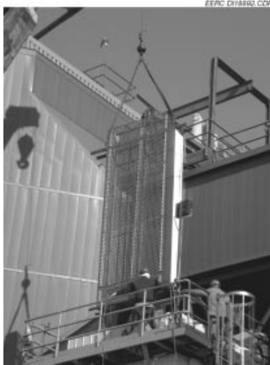
Figure 13. Installing the perforated plates in the 9000-acfm ( 255\text{-m}^3/\text{min} ) AHPC at the Big Stone power plant, March 2001.
