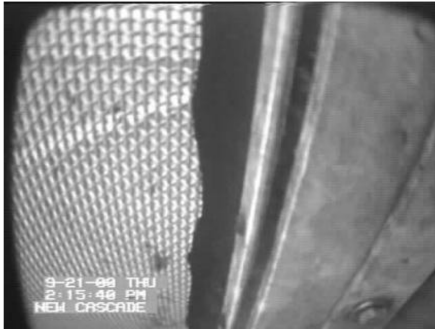
Figure 26. Notched Side Seal on Screen 8 at the New Cascade Site, 9/21/00
