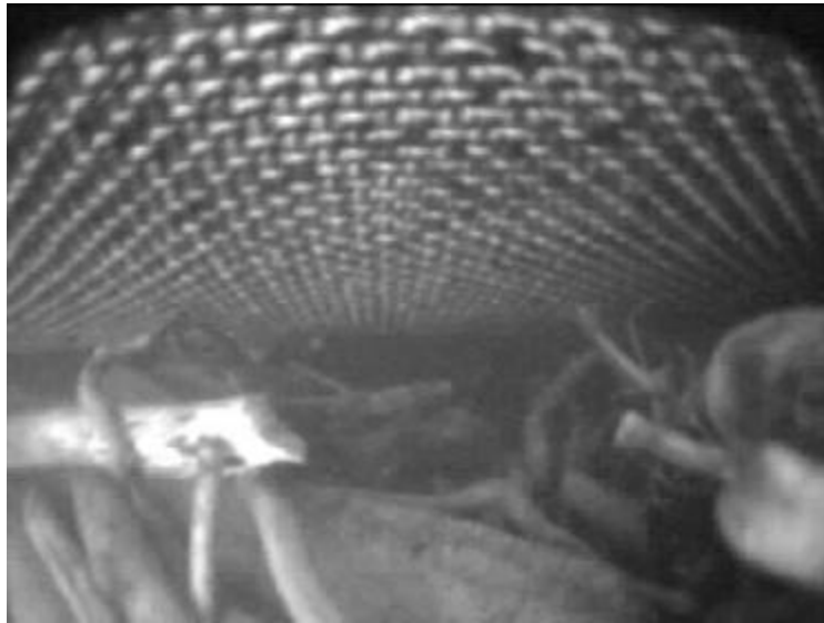
Figure 6. Woody Debris in Front of the Bottom Seal of Screen Number 1 at Bachelor-Hatton on 5/25/00
