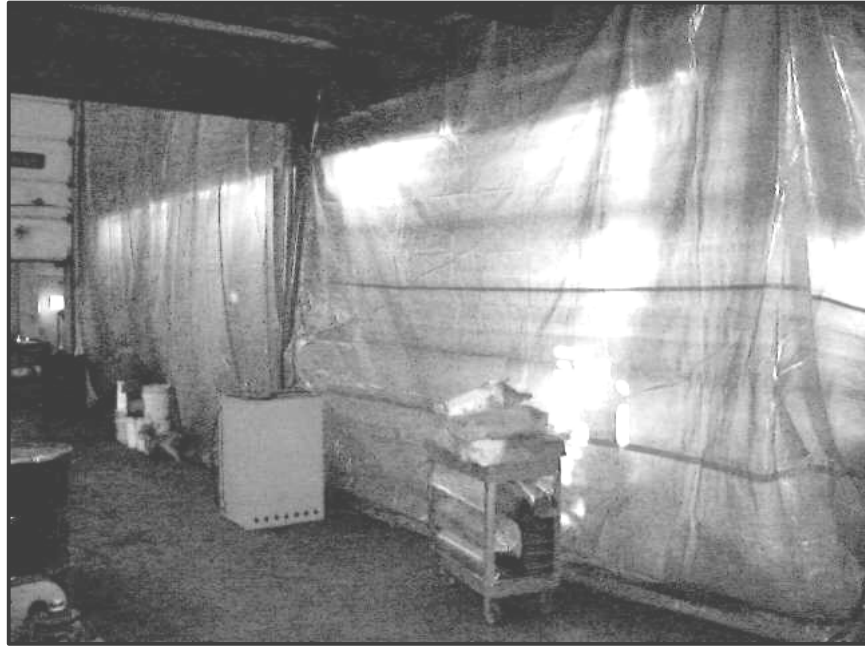
Figure 1. Plastic safety curtains used to restrict airborne dust in the testing facility.
