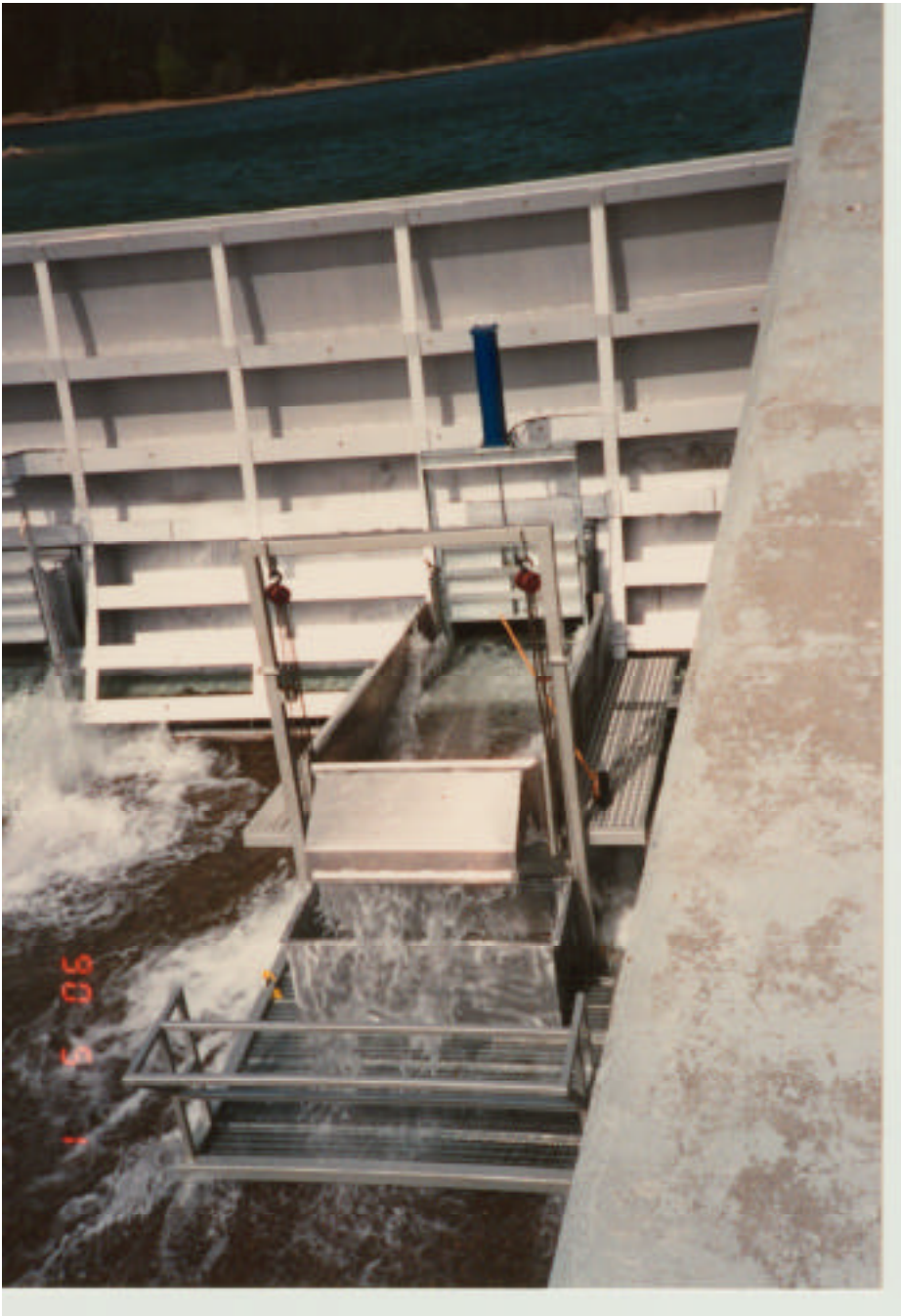
Figure 8. Inclined plane fish sampling trap at radial gates at spillway of Cle Elum dam.
