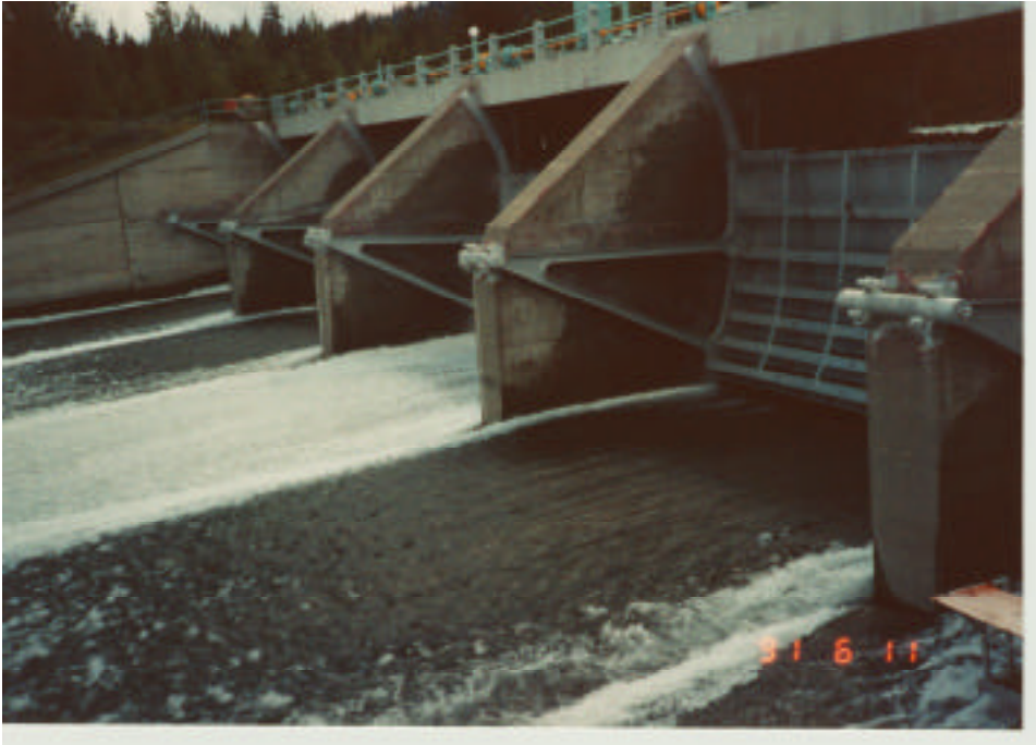
Figure 7. Radial discharge gates at Cle Elum dam.
