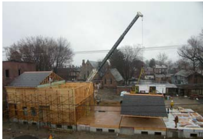
Figure 9. Lifting the roofs into position
