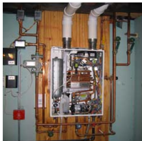
Figure 19. Installed combination boiler
