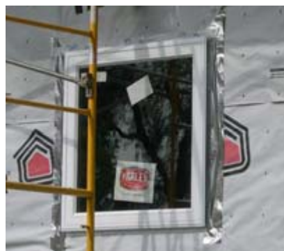
Figure 11. Window installed and flashed
